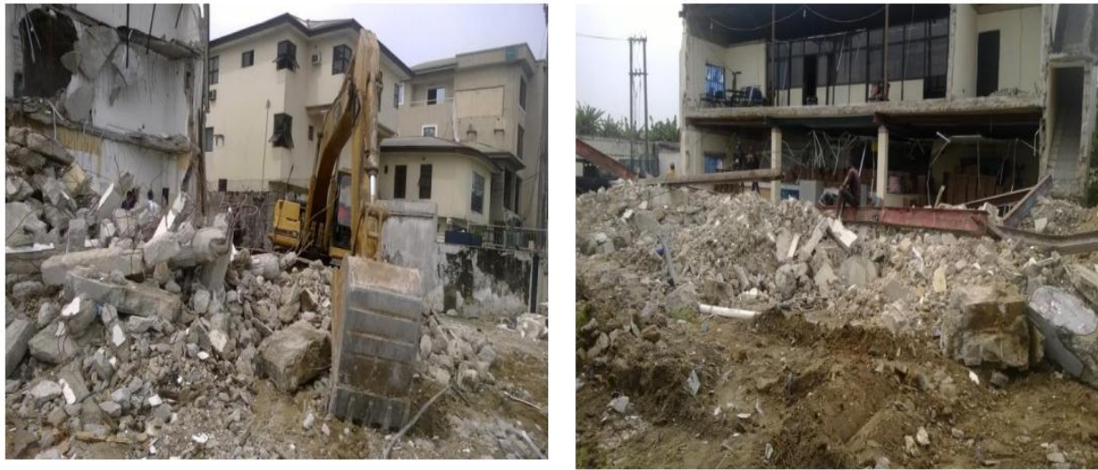
Fig. 2: Demolition Waste Along Trans-Amadi, Port Harcourt, Nigeria (Otoko, 2014)
